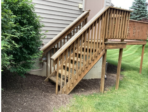
Staircase to utility room
