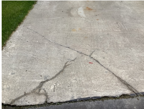
Driveway cracks
