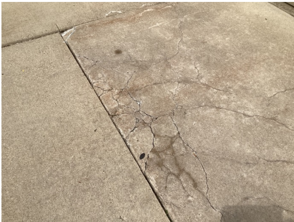
Driveway cracks
