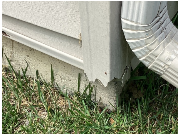
Siding damage
