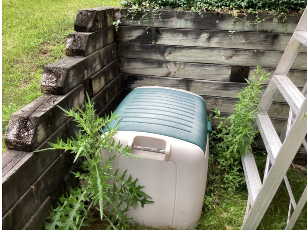
Timber retaining wall
