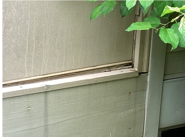
Frame deterioration
