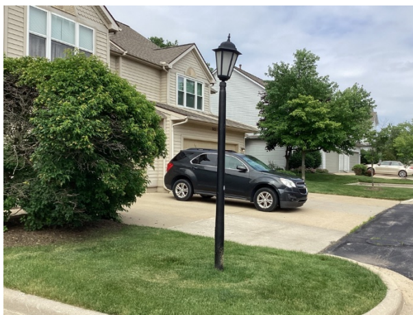
Light pole and fixture - note fixture damage
