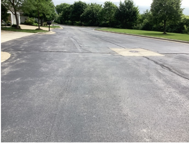
Asphalt pavement street overview
