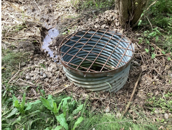
Drainage structure surrounded by stones and vegetation
