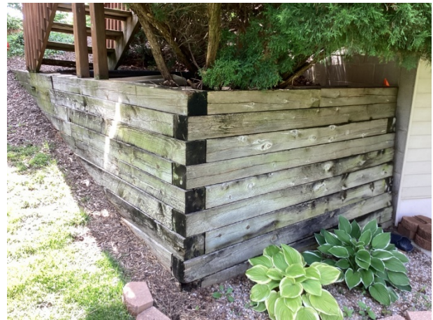
Timber retaining wall
