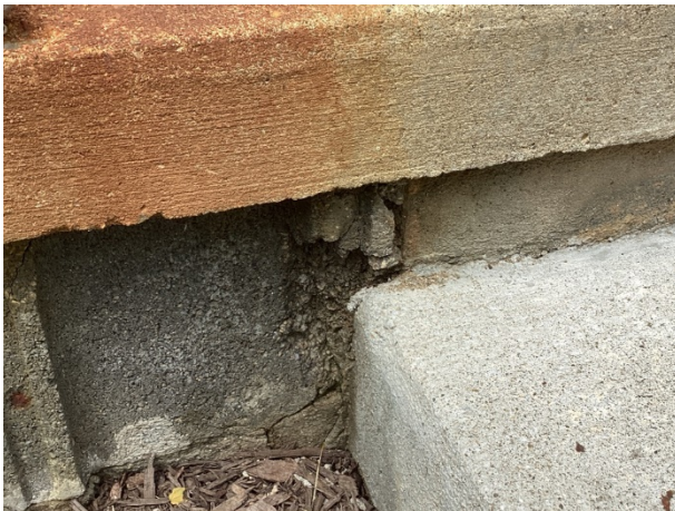
Concrete spalling
