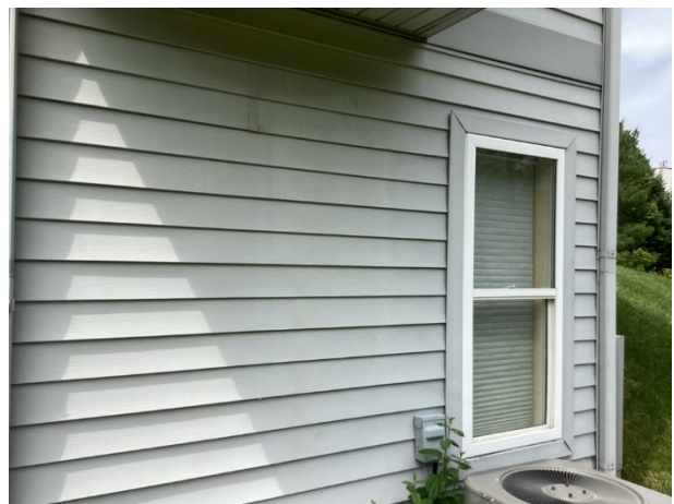
Vinyl siding overview
