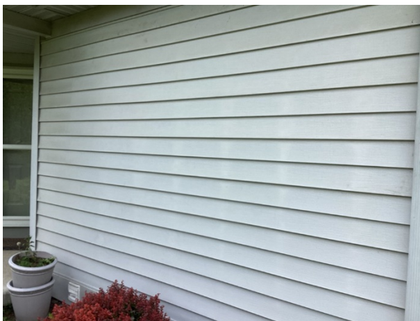
Vinyl siding overview
